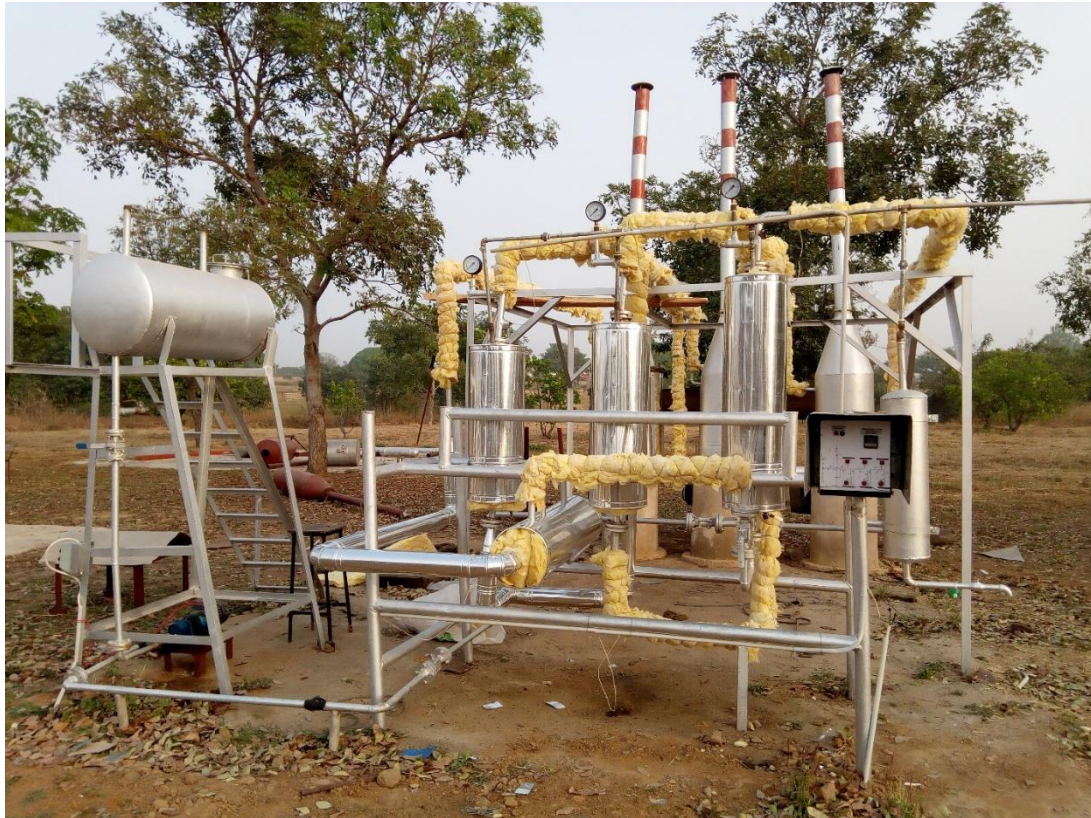
Plate 5: Cladding and Lagging
