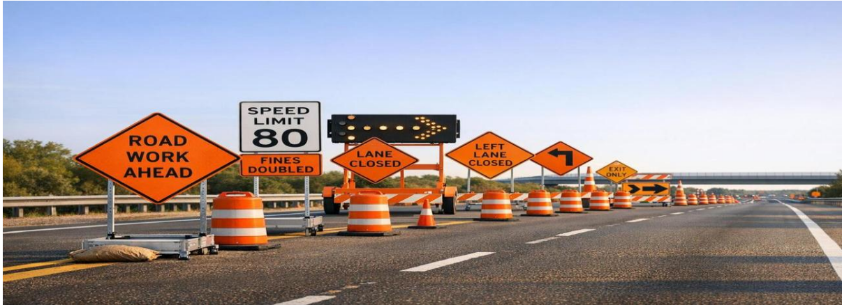
Plate 2: Typical Highway Construction Work Zone for Advance Warning Signs, Channelizing Devices, Barriers, and the Work Area.
