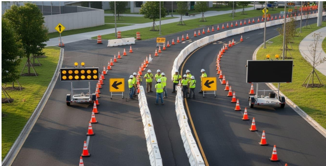
Plate 1: Typical Highway Construction Work
